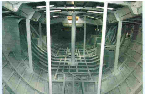
The hull and deck structurally complete, ready for fit-out
